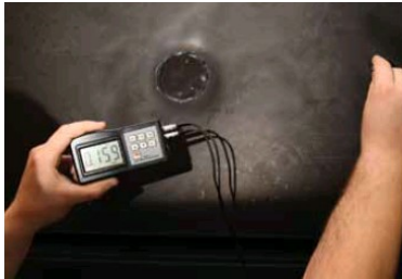
Encasement Wall Thickness Test
